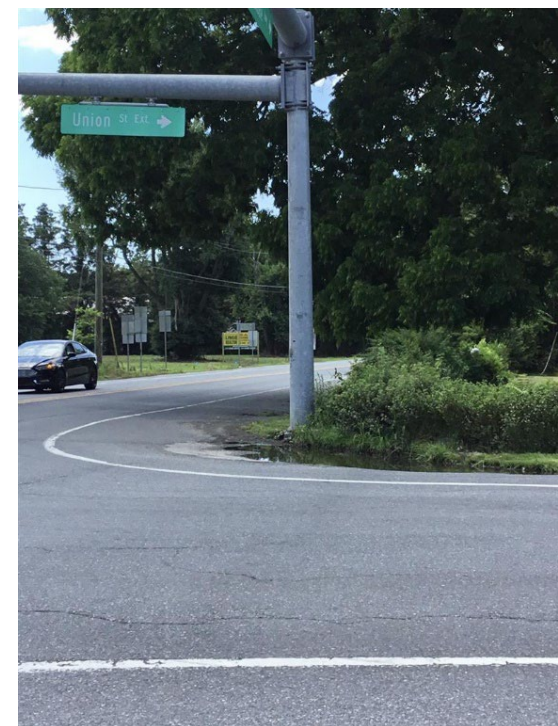
Water ponding on NW corner
